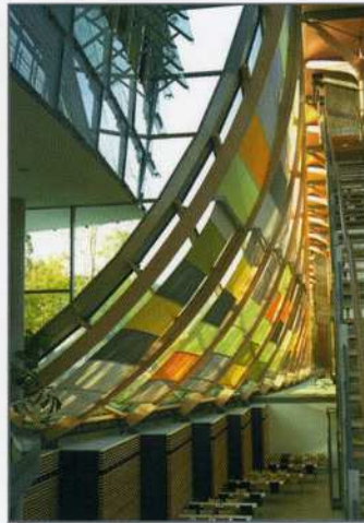
Offices in Landshut - Germany
